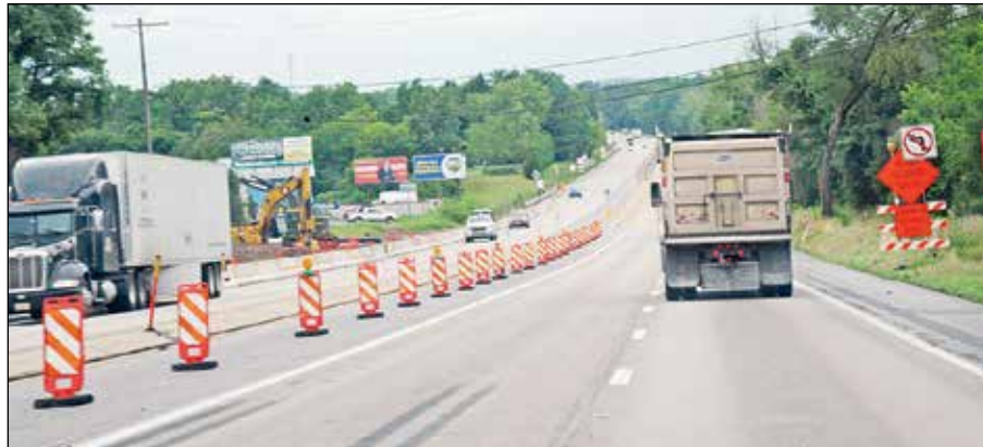
Since mid-July, this stretch of U.S. Route 15 near Franklin Church, Cabin Hollow, and Hickory roads is under construction to include jug handles and longer acceleration and deceleration ramps to eventually make travel on the highway safer.
